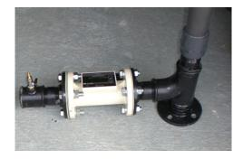
The assembled stack is now over 2.5m above ground level. As this purge system guarantees meeting the velocity requirements of UP/1 there is no need for a flame trap. If the velocity falls below that in UP/1; STOP the purge and investigate.
